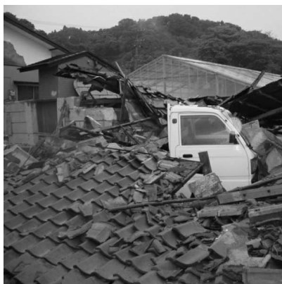
Damage from the Miyagi earthquake photo courtesy Yamato Town
